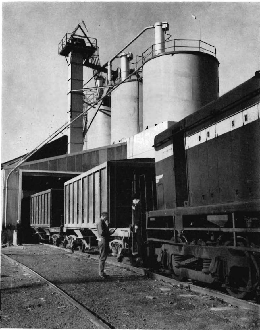
Bulk cement wagons being placed in position for unloading at a metropolitan siding.
