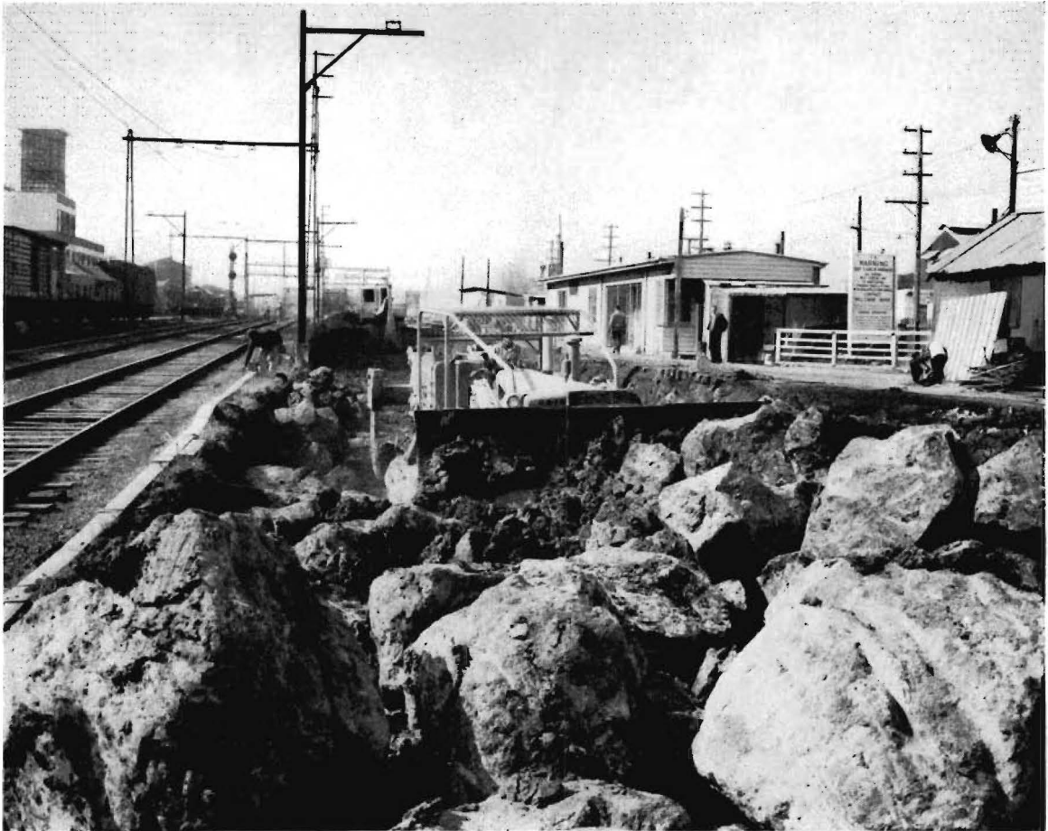
Removal of boulders during excavation work for the Richmond-Burnley track quadruplication.
