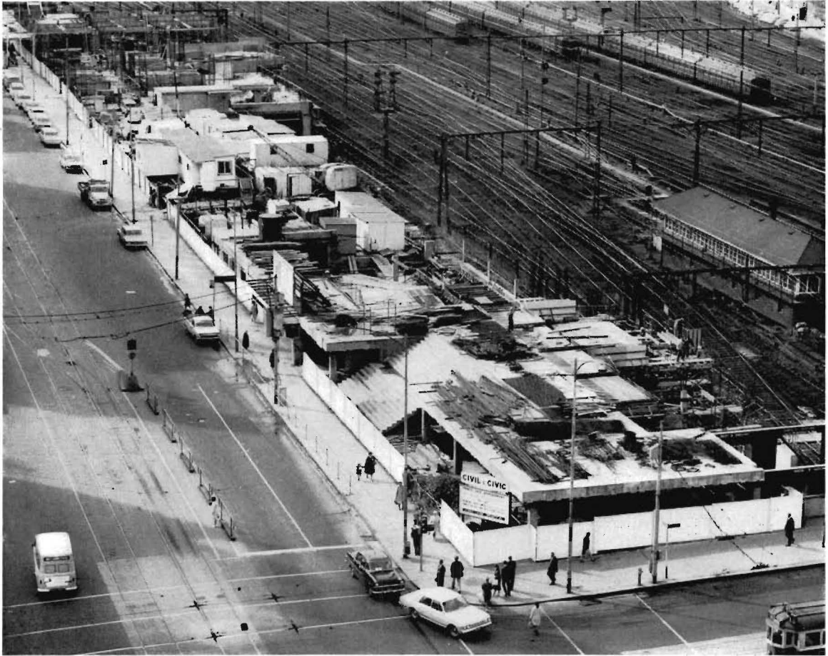
Progress of work on Princes Gate Development project.
