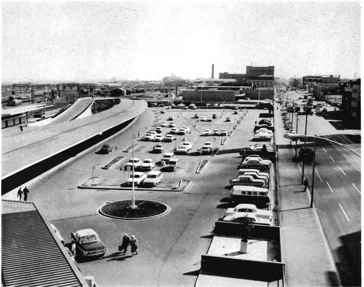
Spencer Street Station Car Park.
