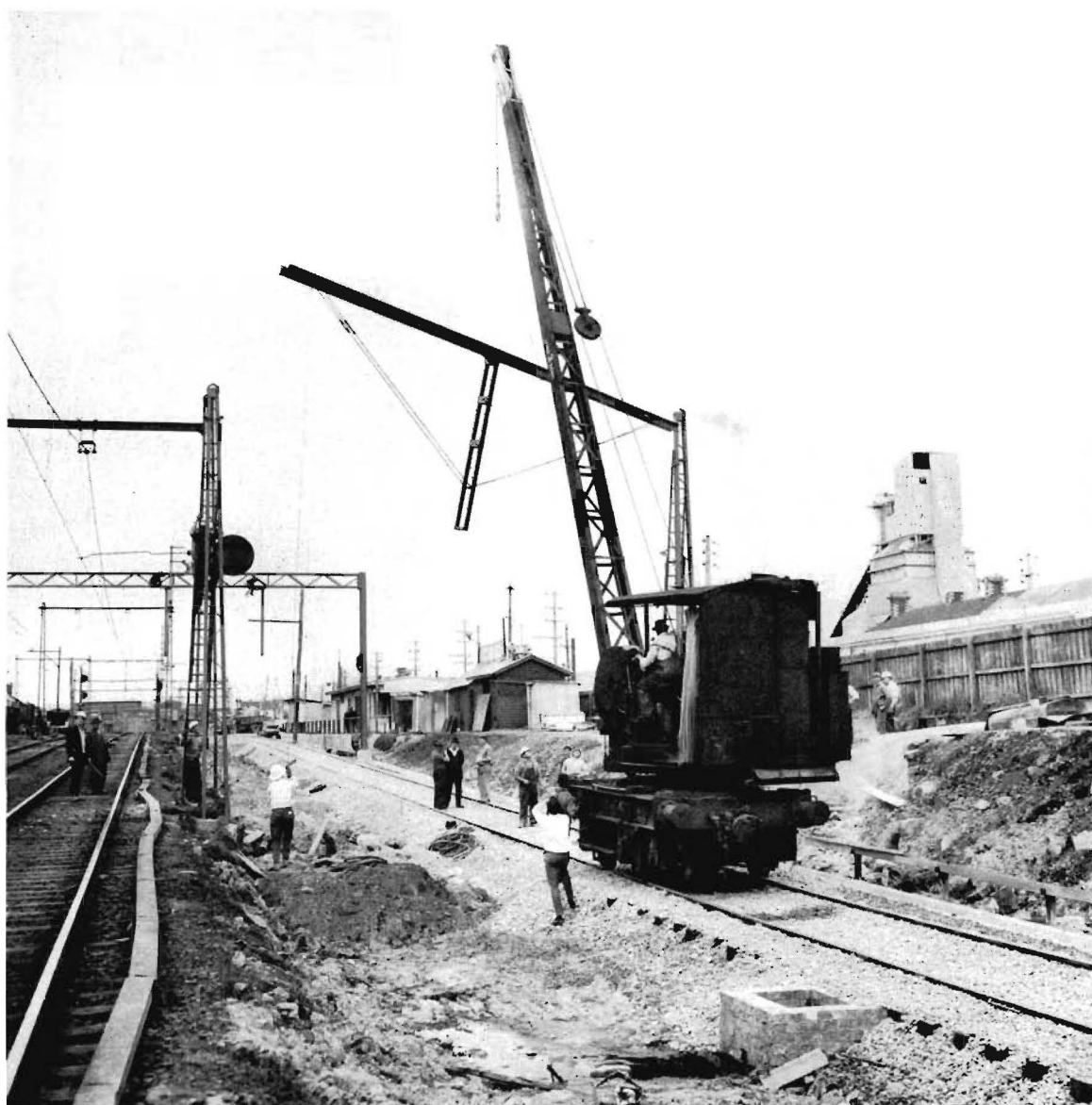
Erection of overhead structures between Richmond and Burnley.
