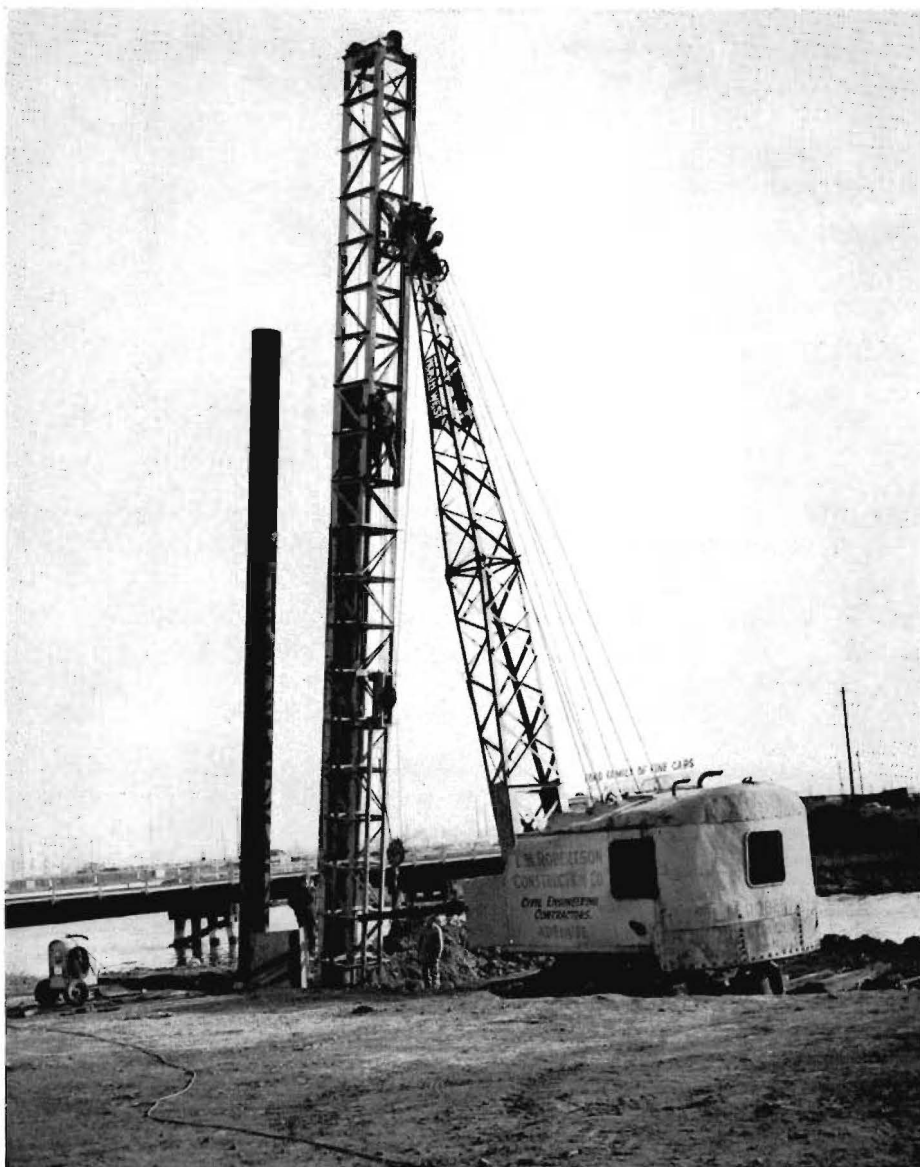
Driving piles for new bridge over canal at West Melbourne.
